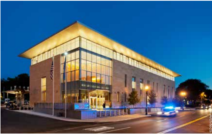
▲ Dudley Square Police Station in Boston.
